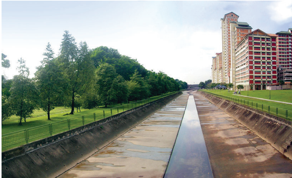
Technical waterway before redesign – sealed canal in Bishan Park before reconstruction.
